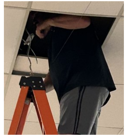
James Russum installing new lights in the hall on 7-3-26.
